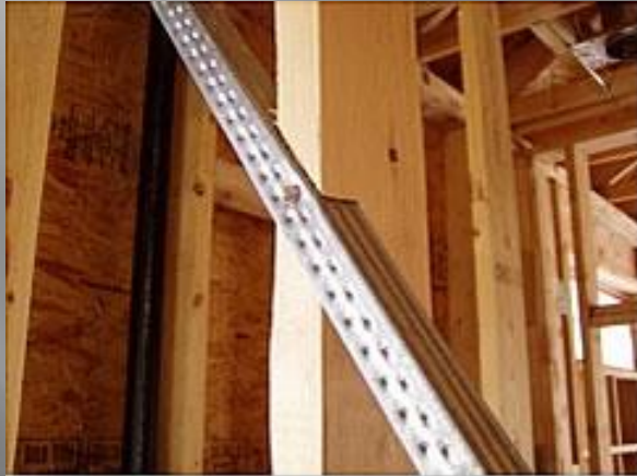
Bracing installed in a saw kerf
