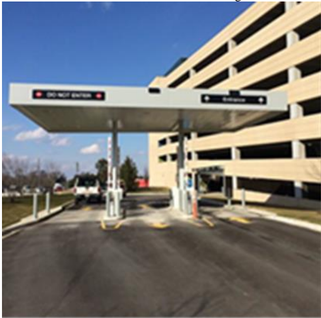
Picture: Entrance to Hill Farms Parking Structure
