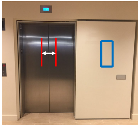
For an elevator with center-opening hoistway doors, a solid smoke door must have a vision panel as shown in the location that corresponds to the first one-fourth of the hoistway door's travel when opening.
