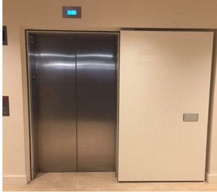
A solid door without a vision panel will not meet A17.1, 2.11.6.3 (d).
