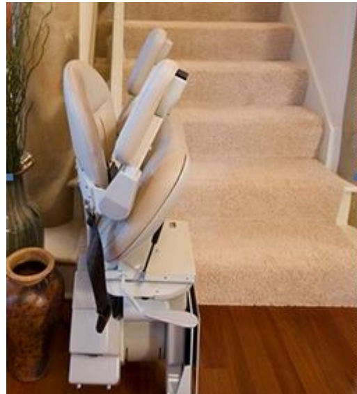
Stairway chairlift in Folded position, NOT to be used for measuring remaining stairway width
