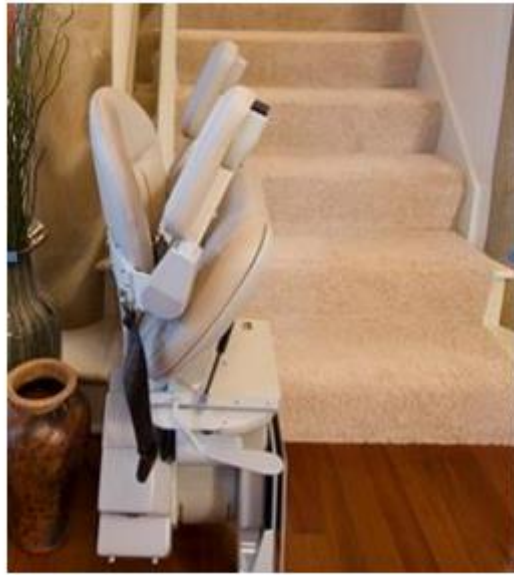
Stairway chairlift in the Folded position, NOT to be used for measuring remaining stairway width
