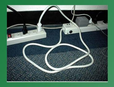
11.1.7.3 Extension cords shall be maintained in good condition without splices, deterioration, or damage.
