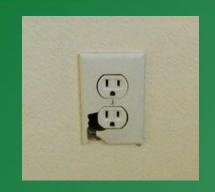
11.1.10 Covers All panelboard and switchboard, pull boxes, junction boxes, switches, receptacles, and conduit bodies shall be provided with covers comparable with the box or conduit body construction and suitable for the conditions of use.
