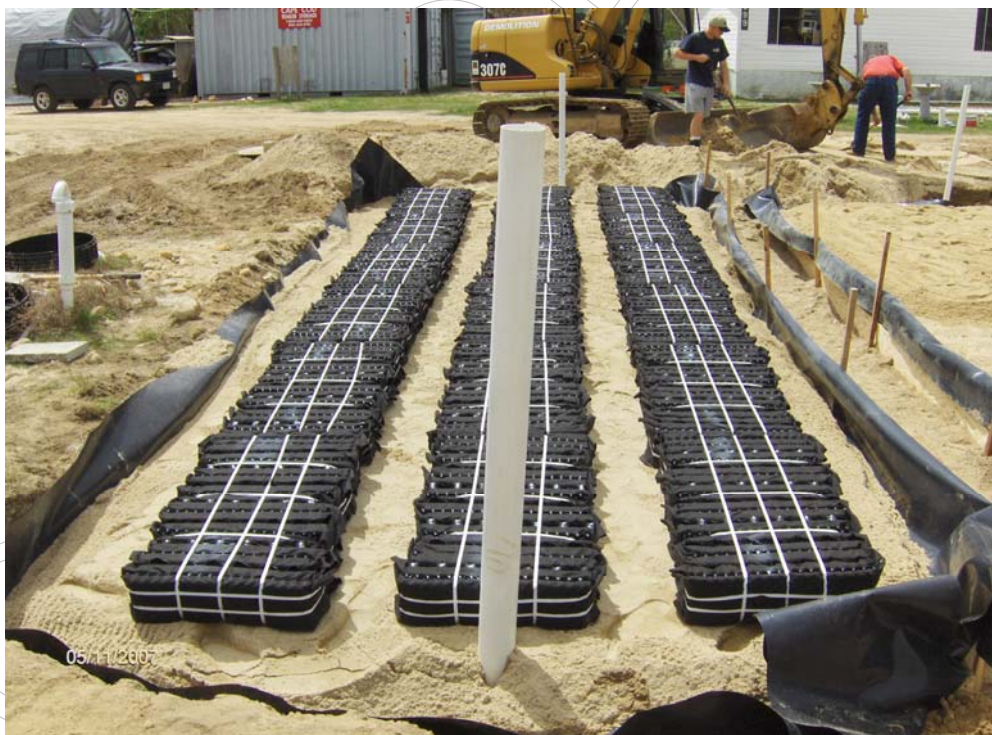
Figure 5. Eljen GSF modules are placed on the prepared test cell.
