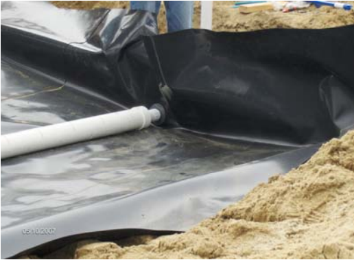
Figure 2. The four-inch underdrain is connected to a watertight bulkhead fitting. The drain pipe on the outside fitting is directed into a distribution box for sample collection.
