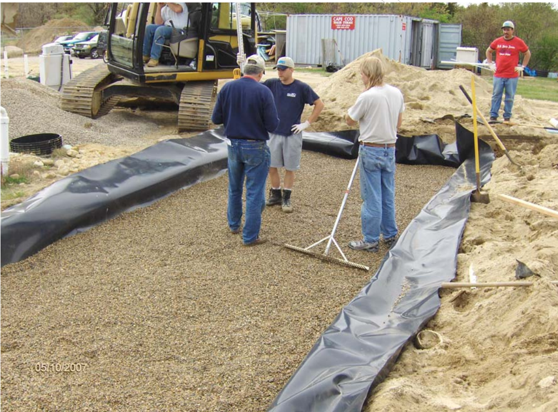
Figure 3. Two to six inches (six inches in the center low point to two inches on the upslope of each side) of washed 1/8 inch aggregate is placed at the bottom of the liner to allow for free flow of percolate toward the collection drain.
