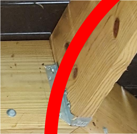
Flange bent for angle of deck
