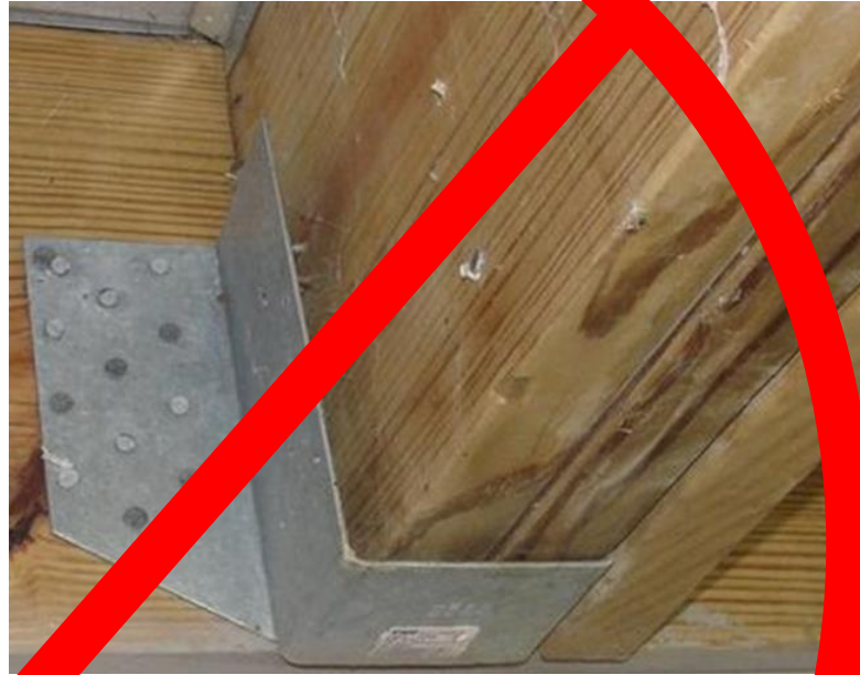
3 ply beam, 2 ply hanger
