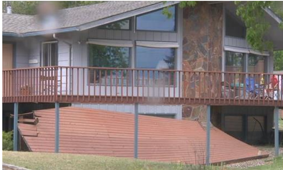
August 2, 2016 Roughly 40 people on deck Fell about 10 Feet
